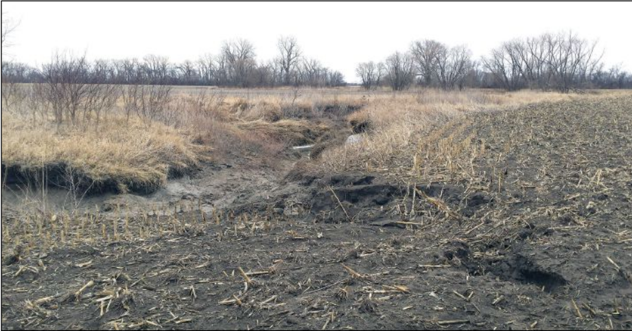
Initial stream bank erosion.
